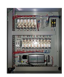
A controls system manages the distribution and cleanliness of the water within the bladder. To extract water, a pump is utilized and activated when called by the user. Sensors placed within the system sanitize the water through a UV light filter, in addition to monitoring the amount of water in the bladder.
