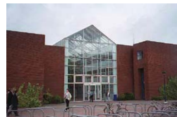
Grattan Building, DCU
